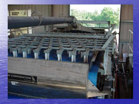
Digested sludge is mixed with polymer and applied to the belt press.
