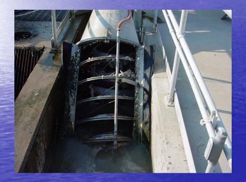
After wastewater is pumped into the Headworks of the plant, it will flow through a fine screen to remove large particles of waste.
