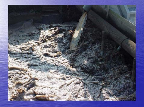
As mentioned previously, constant reproduction will force an operator to dispose of or "waste" some of the "bugs" in the process in order to keep the food to microorganism ratio at a sustainable level.
